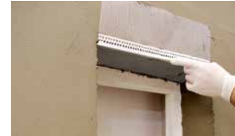
Installing the Kale Meshed PVC Corner Profile on window corners.
