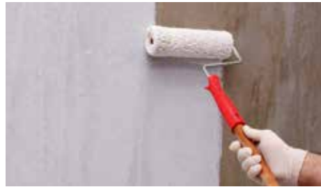
Priming the surface with Silastar.
