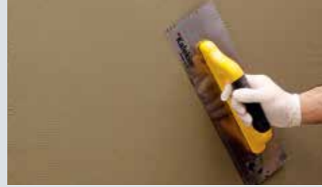
Application of 2nd plaster coat.
