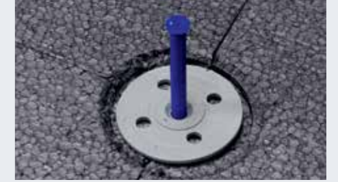
Anchor is placed and the pin is removed.
