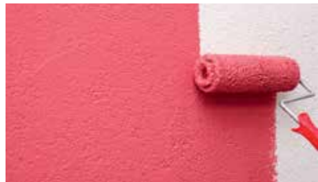
Kale Exterior Paint application on Minart
