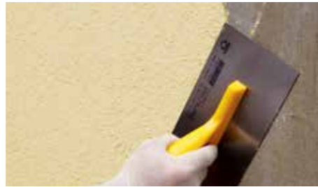
Decorative coatings are applied on the surface using a trowel. Thickness, of the application changes depending on the plaster type.
