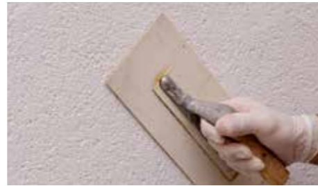
Texture is formed by glazing the coatings on their surface with a plastic trowel before they dry. Since Minart is mineral based, it must necessarily be primed with Kale Silastar and painted with water based Kale Exterior Paints after it dries.
