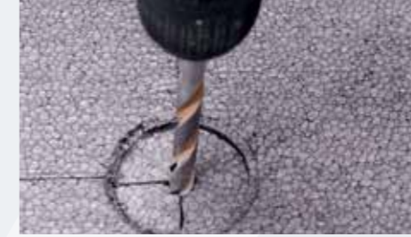
Anchor point is drilled.
