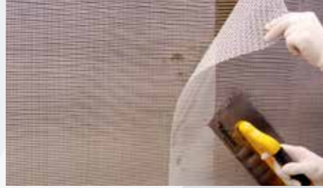
10 cm overlapped application of reinforcement mesh.
