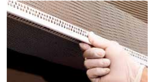
Installing the Kale Meshed PVC Edging Profile.
