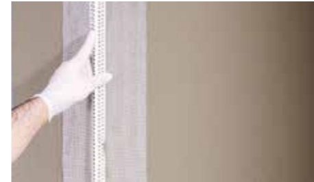
Installing the Kale Meshed PVC Corner Profile.
